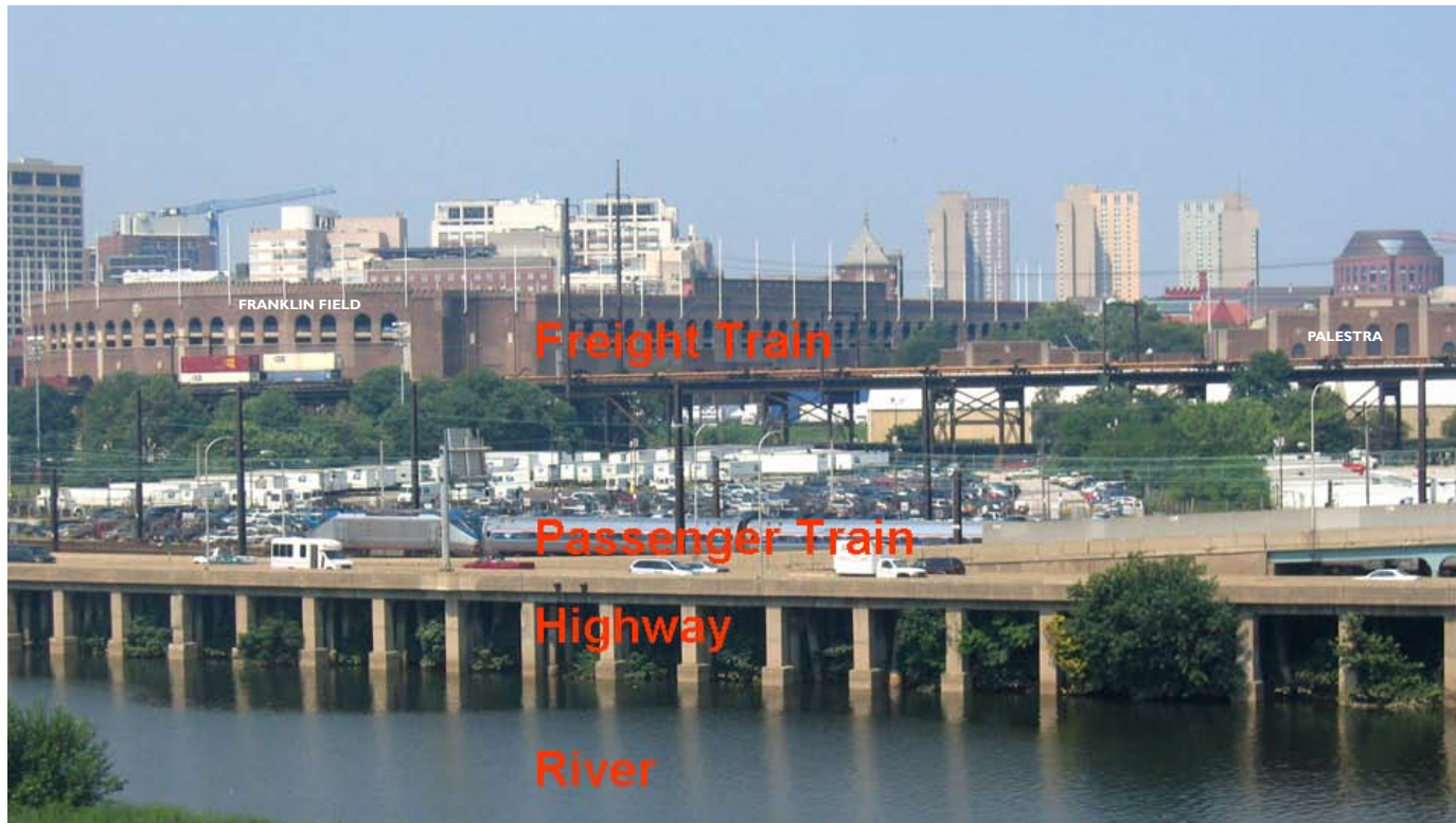
Photo of the east campus area as viewed from the east side of the river. The photo illustrates both the complexity of the infrastructure and the iconic quality of Franklin Field and the Palestra.
