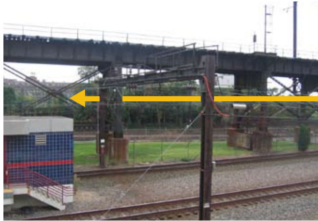
Proposed crossing point of the Research Bridge over the rail lines and under the Highline in the area of University City Station
