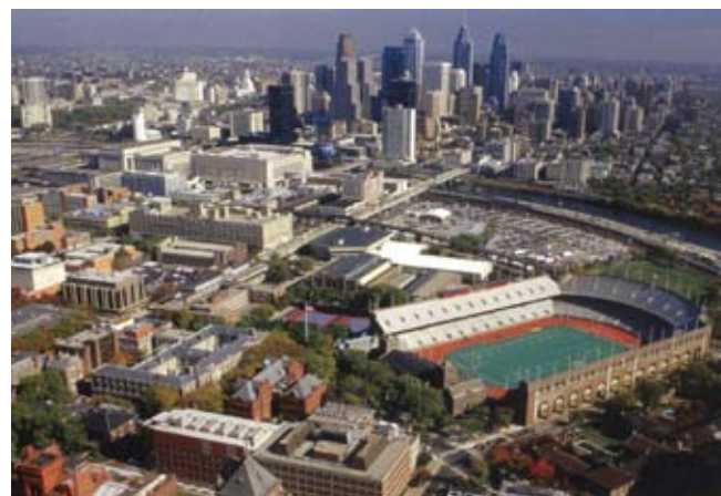
View of the east campus area looking east
