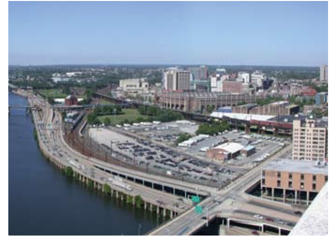
View of the east campus area with the surface parking area of the postal lands in the foreground.
