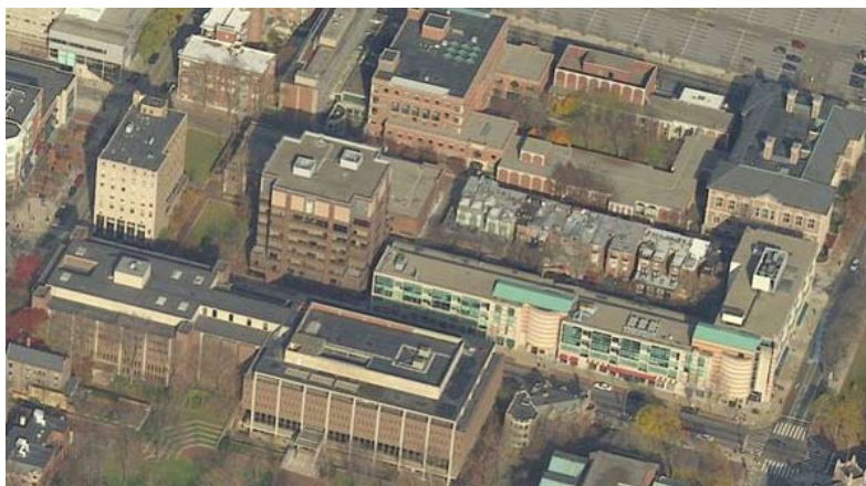
Existing Conditions at 3400 Walnut
