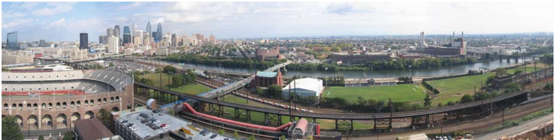
View of existing conditions in the east campus area illustrating the South Street Bridge, Highline, University City SEPTA Station, and the Amtrak corridor.
