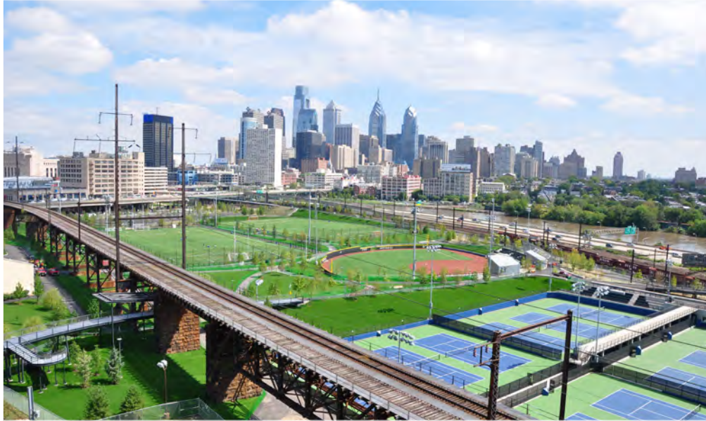
View Northeast toward Center City Philadelphia
