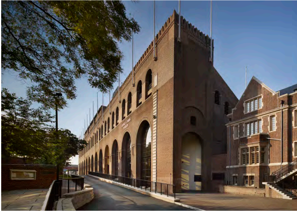
Porous pavements at Weiss Pavilion
